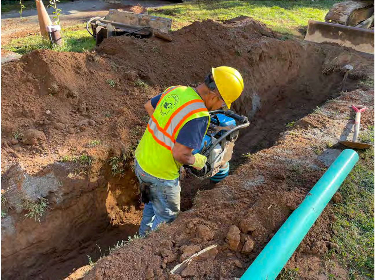
Picture 2: Ludlow compacting backfill with a jumping jack in the trench they excavated for the installation of a 1" copper water service line at the 298 Main Street residence. View to the southwest.
