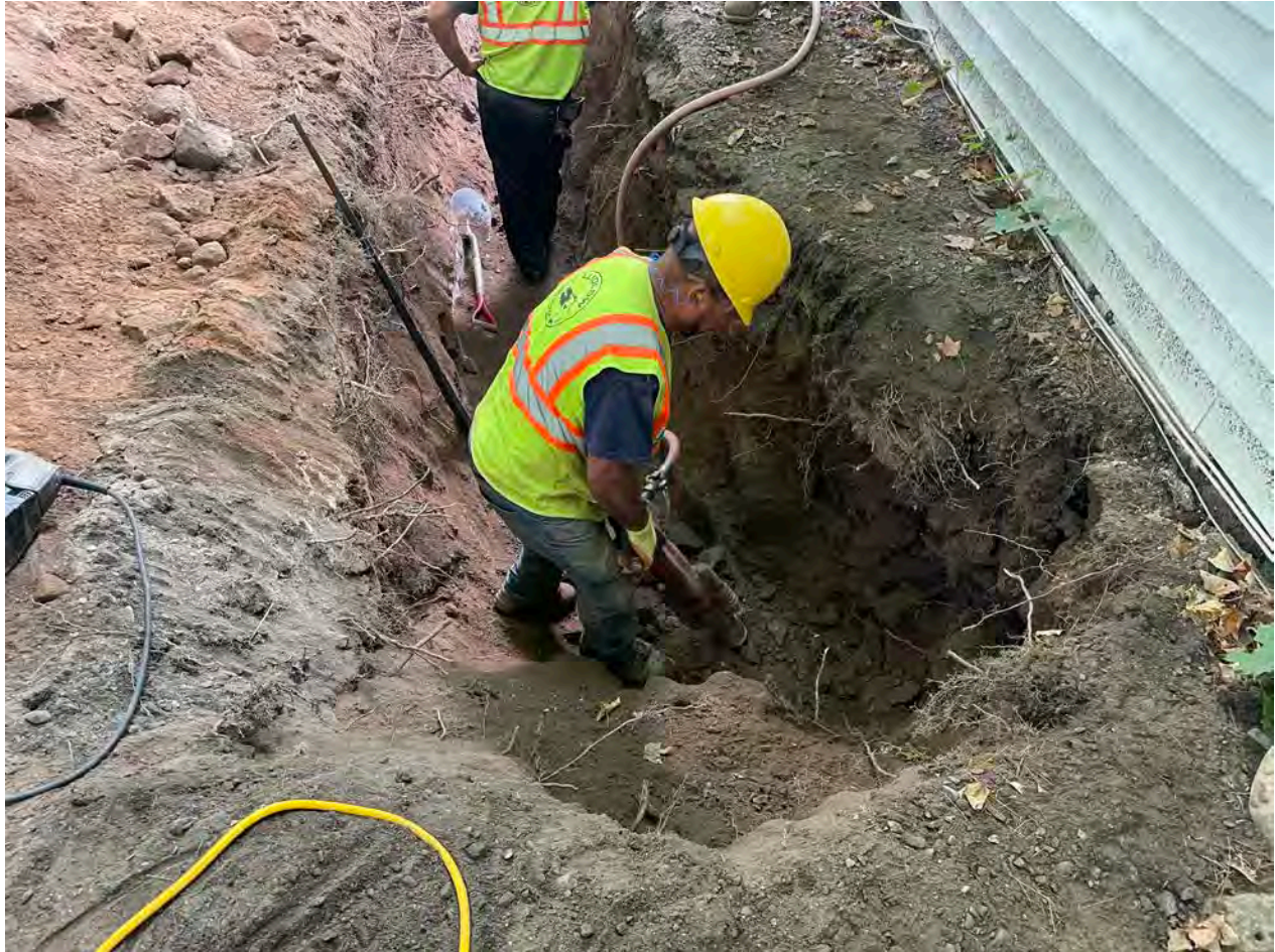
Picture 7: Ludlow using a jackhammer to break up bedrock they encountered when excavating a trench on the north side of the 312 Main Street residence for the installation of a 1" copper water service line. View to the east.
