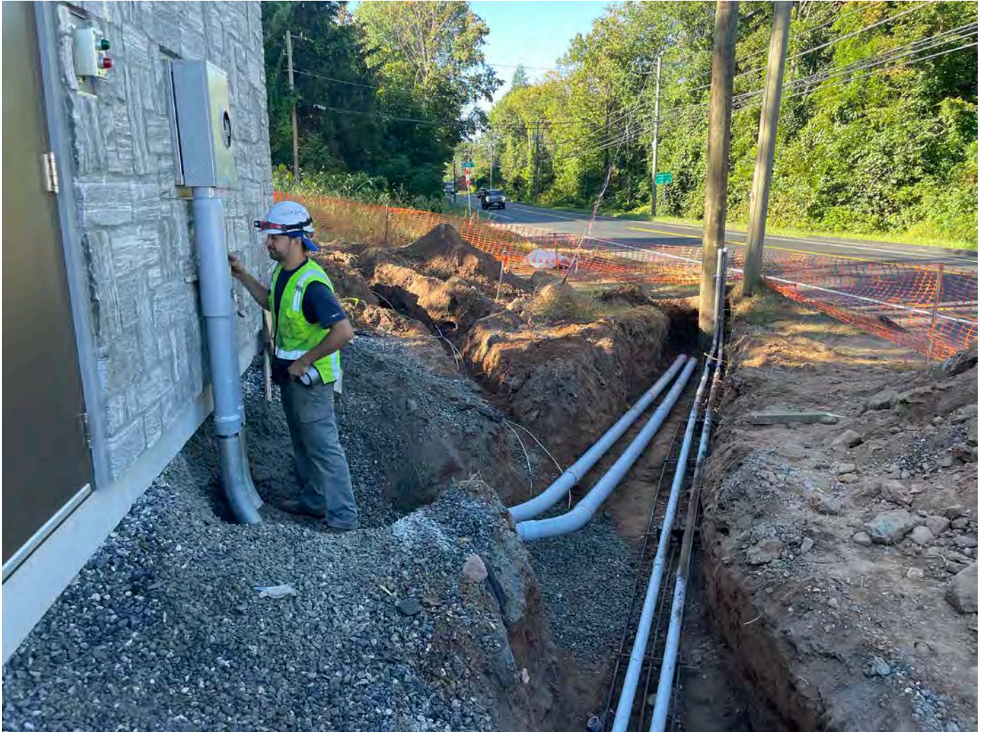
Picture 4: A&R Electrical installing conduits at the meter station building located at Station 124+80 S. Main St. Middletown. View to the southwest.
