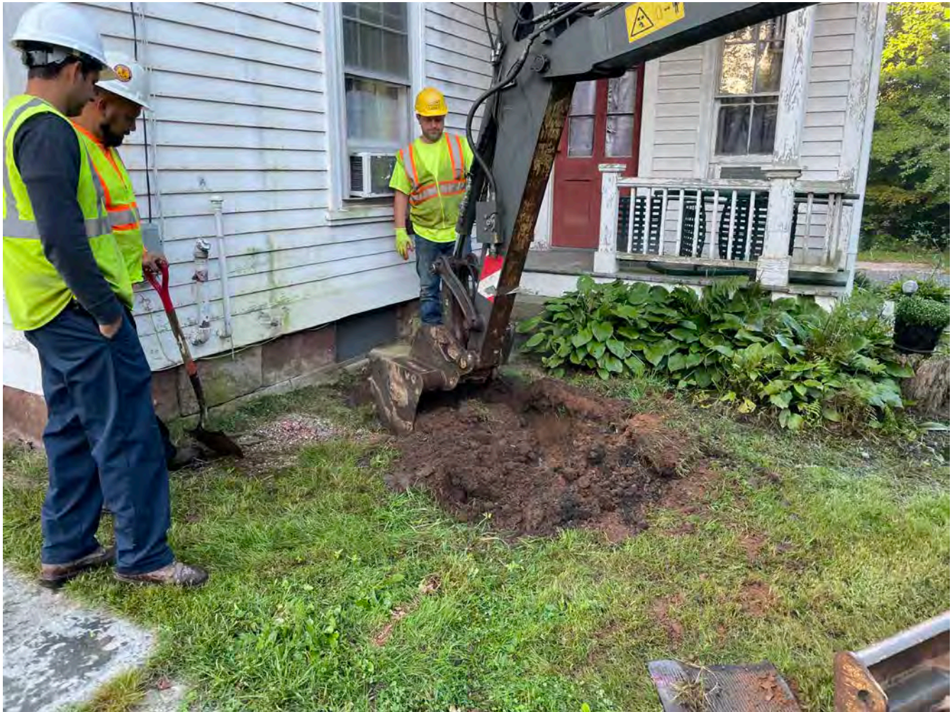
Picture 1: Ludlow beginning to excavate at the northeast corner of the 298 Main Street, Durham, residence on the north side of the home. View to the southwest.
