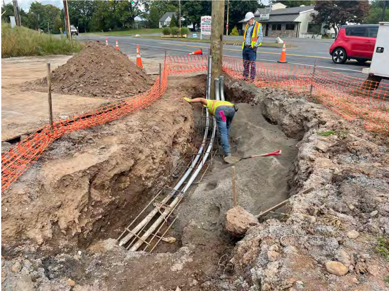
Picture 8: Ludlow placing rebar under and over the 2" PVC conduits coming off one of the recently installed poles at the booster station located at Station 750+63 S. Main St., Middletown. View to the northeast.
