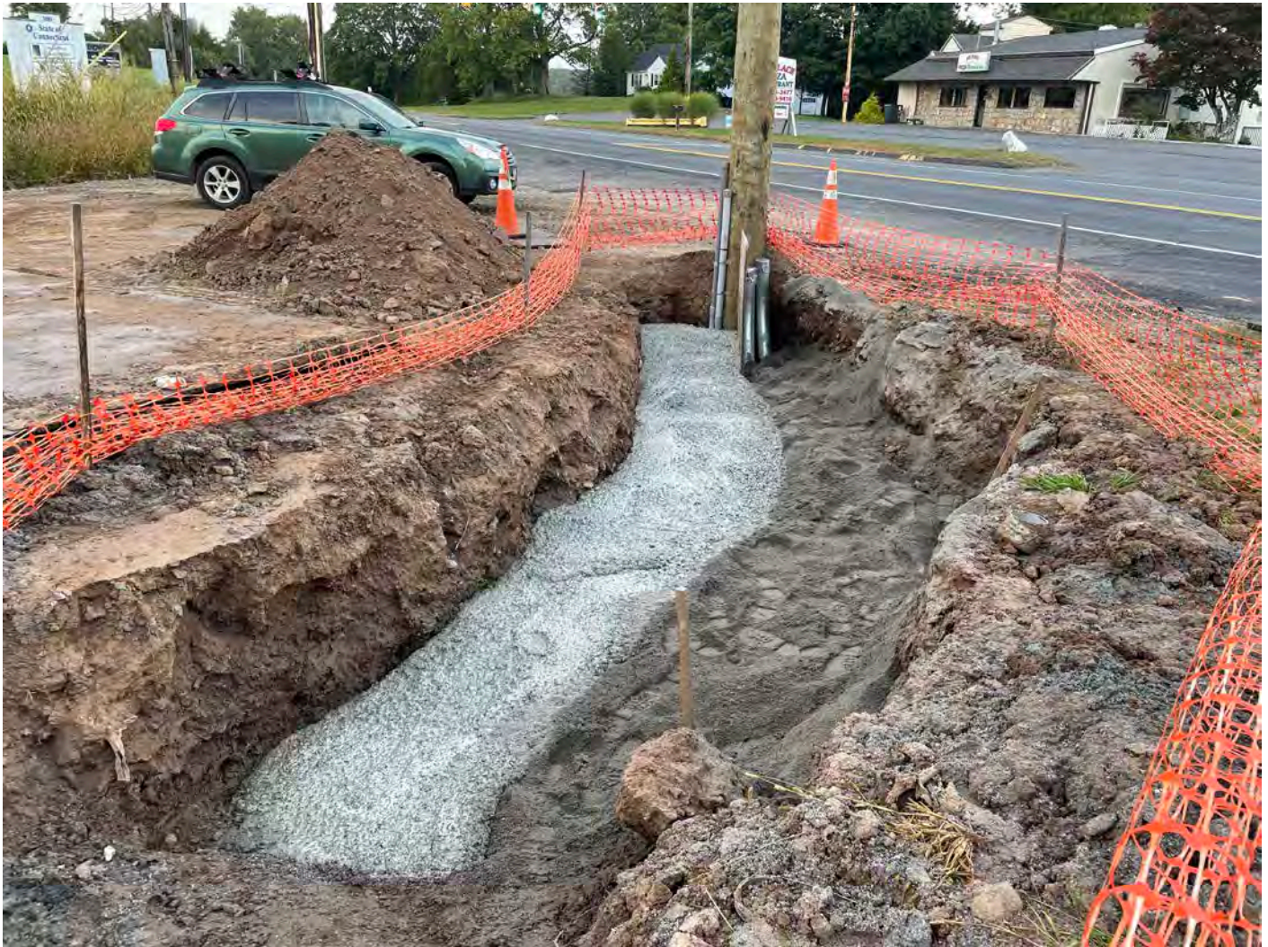
Picture 12: View of the concrete that was placed over PVC conduits at the booster station located at Station 750+63 S. Main St. Middletown. View to the northeast.
