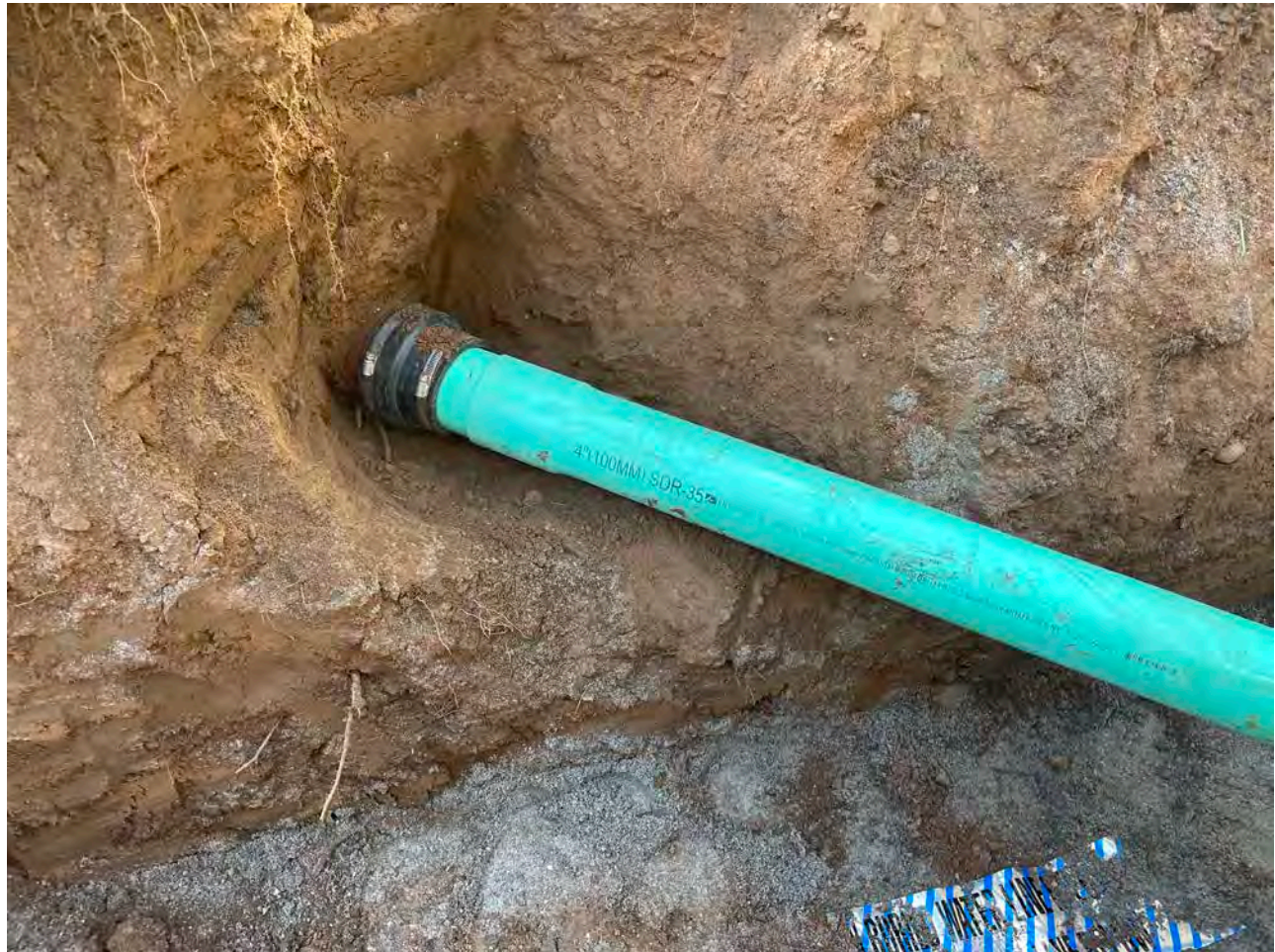
Picture 3: 4" PVC and Fernco boot used to repair a clay drain line that was broken during the installation of a 1" copper water service line at the 298 Main Street residence.
