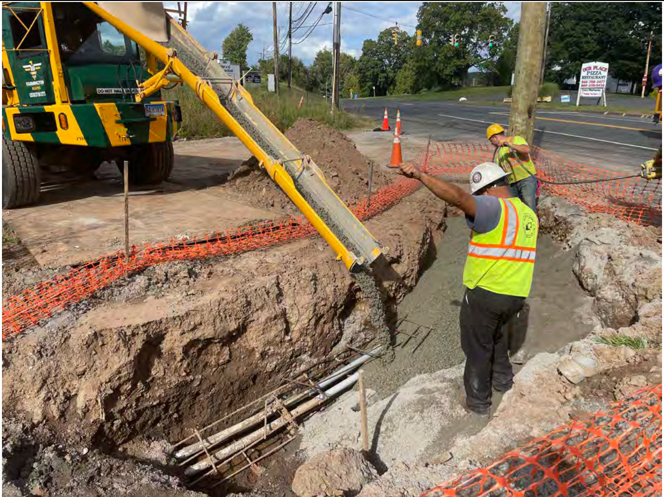
Picture 9: Ludlow directing the placement of 4000 PSI concrete over the 2” PVC conduits coming off one of the recently installed poles at the booster station located at Station 750+63 S. Main St. Middletown. View to the northeast.
