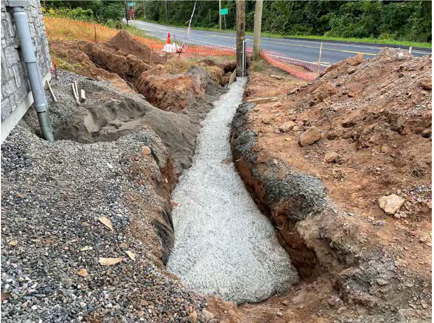
Picture 11: View of the concrete that was placed over PVC conduits at the water meter building located at Station 124+80 S. Main St. Middletown. View to the south.
