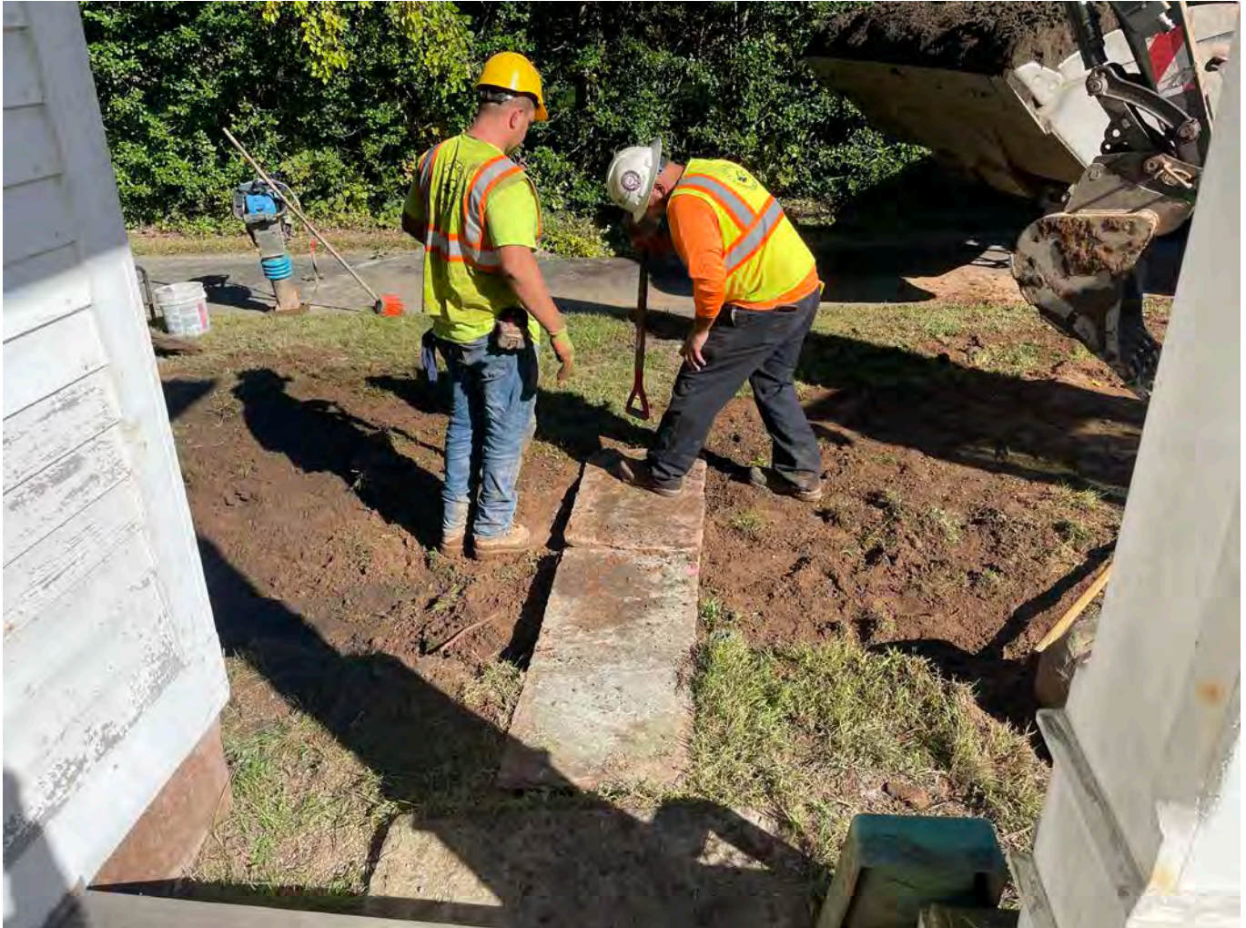
Picture 5: Ludlow replacing pavers for the walkway at the 298 Main Street residence after the installation of a 1" copper water service line. View to the north.
