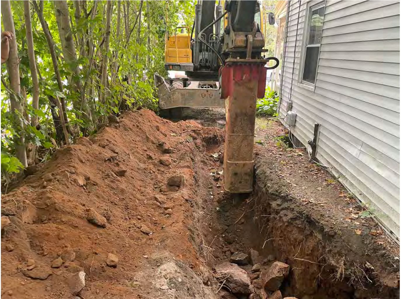
Picture 6: Ludlow using a hammer to break up bedrock they encountered when excavating a trench on the north side of the 312 Main Street residence for the installation of a 1” copper water service line. View to the east.
